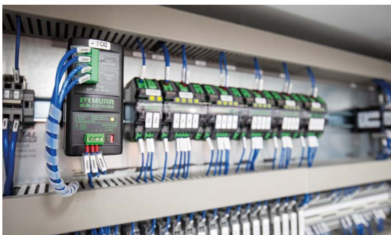
A view into the control cabinet with MB Cap buffer module
